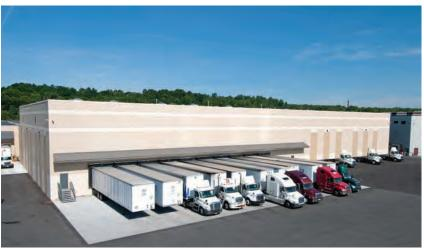
Decrescente Distributing Company selected BBL to construct an addition, as well as, renovate their existing warehouse. The exterior wall system is constructed of insulated precast concrete wall panels. The interior fit-up included creating a 20,000 sf cooler within the existing building. The facility is the central hub of DeCrescente's operations and remained operational during all phases of construction.
