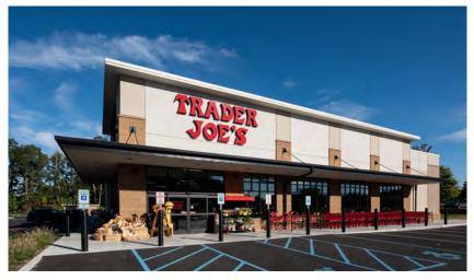
BBL provided site work and shell construction for this 12,500 square foot retail building. Work included concrete foundations, structural steel, metal framing, sheathing, roofing, masonry, EIFS, MEPs, storefronts and autodoors. The building is occupied by Trader Joe's, a national grocery store offering high end products at everyday prices to the community.
