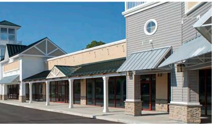
This project included the demolition of two existing structures and the construction of a new 49,613 square foot, one story core and shell building for future retail space. The building consisted of a structural steel framing with a cultured stone and vinyl siding veneer, EPDM roofing for the main building and standing seam metal roof panels over timbered framed canopies at front of building covering the front sidewalk area.
